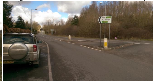
Looking north along Bath Road – the site is to the left
